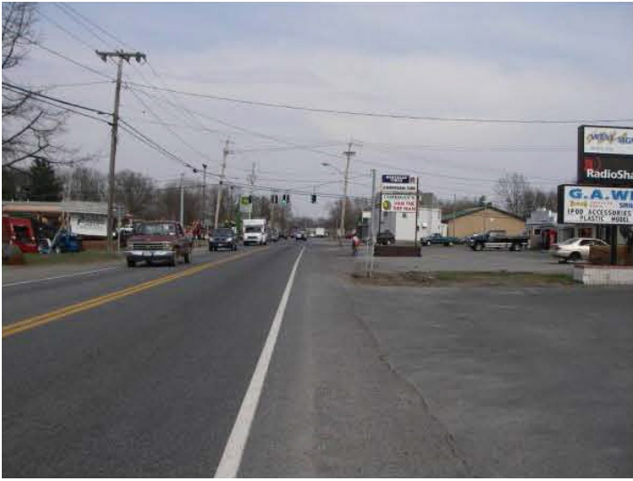
A roadway similar to Boston Street with poorly managed access
