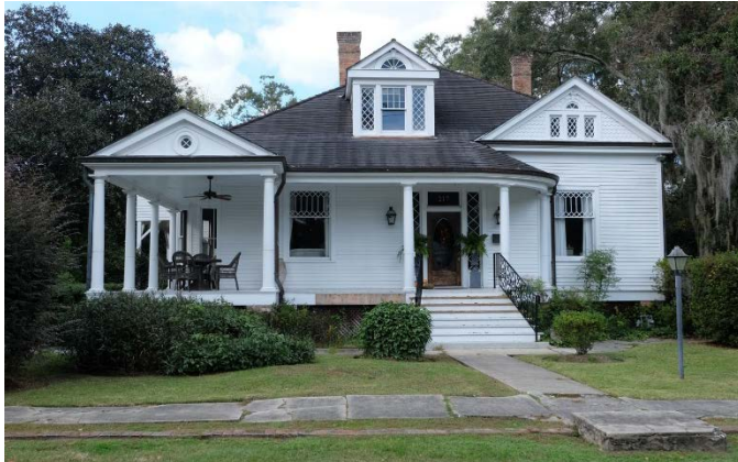
Image 16. Example of a Queen Anne house, 217 South New Hampshire Street, Survey ID #762.
