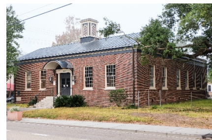
Image 30. Old Covington Post Office, Survey ID #279.
