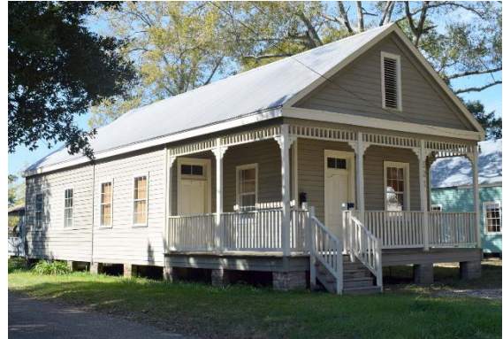
Image 20. A c. 1900 Eastlake/Stick style house at 521 North Florida Street (Survey ID #463A). The resource has sustained alterations, including the replacement of wall cladding, doors, and windows, and enclosure of a portion of the side porch; however, the house retains many character-defining features, such as decorative elements, and replacement materials are compatible.
