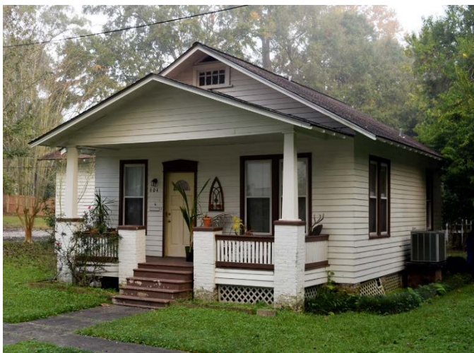
Image 13. Bungalow house, 604 East Independence Street, Survey ID #111.
