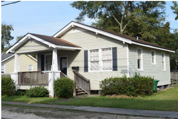
Image 21. A c. 1930 Craftsman bungalow at 430 North Florida Street (Survey ID #424). The wall cladding and porch elements were replaced on this house and shutters were added; however, other important materials and evidence of craftsmanship are extant, and these modifications do not alter the overall appearance of the primary elevation.
