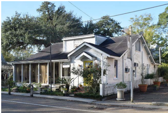
Image 24. A c. 1930 bungalow at 311 Lee Lane (Survey ID #337B). In addition to the replacement of historic materials, the front porch on this resource has been modified from full-width to partial-width, and the resource has been converted from a single-family residence to a commercial specialty store.
