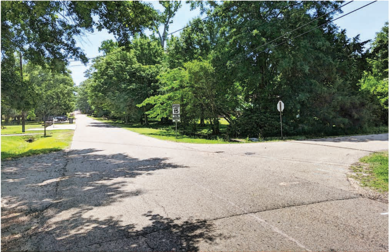
Figure 5.10: Existing Conditions Image - West 17th Avenue and South Harrison Street
